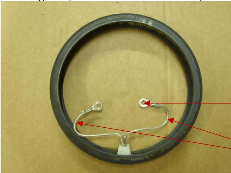
Heating element is fitted with the flat side of the connector terminal facing downwards
